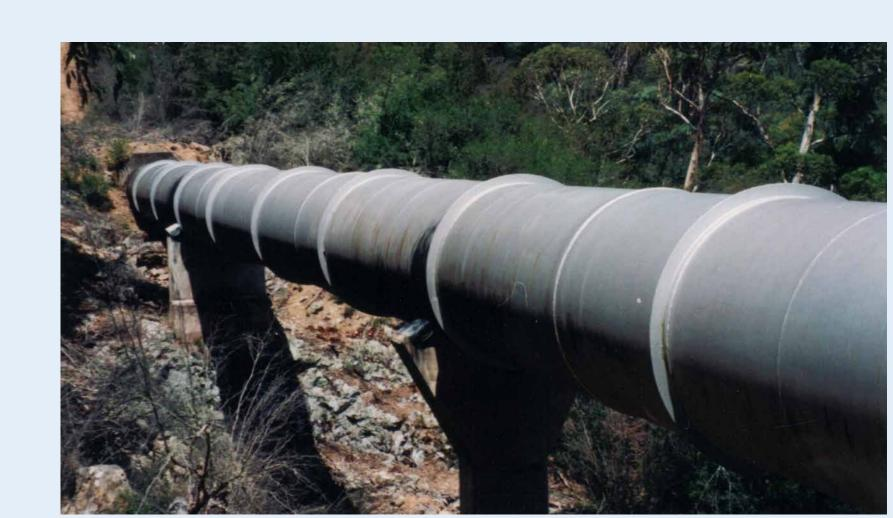
Two trunk feeder mains mostly constructed of Mild Steel and some above ground pipework at Lower Molonglo Sewage Treatment Works
